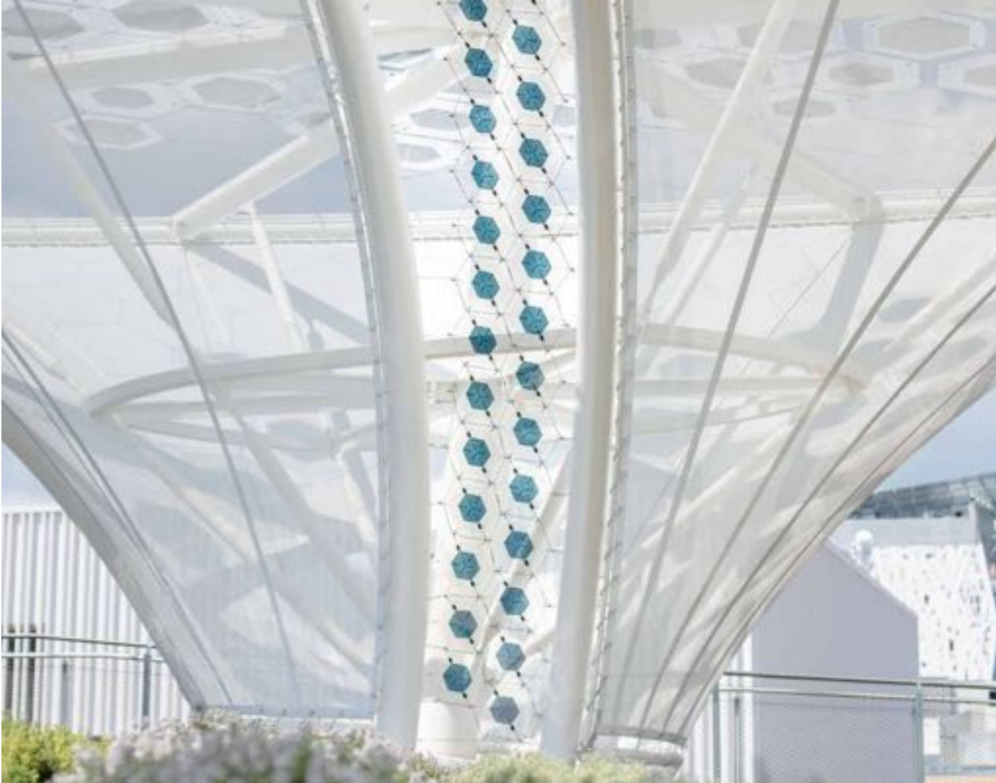
Organic photovoltaic objects on German pavilion at the world exhibition in Milan
